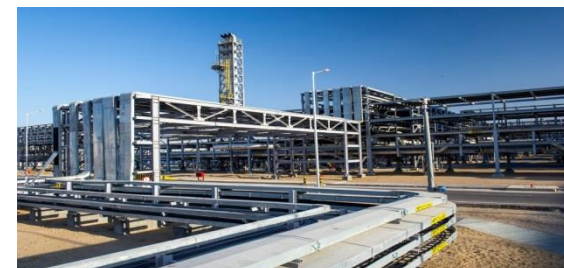
Mangala Processing Terminal
